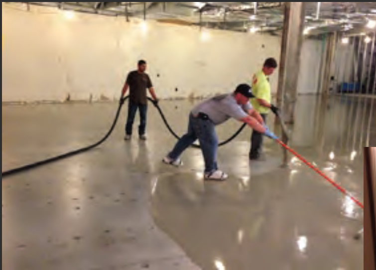
OVERLAY IN PROCESS
