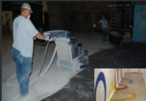
COATING REMOVAL & FLOOR PREP
